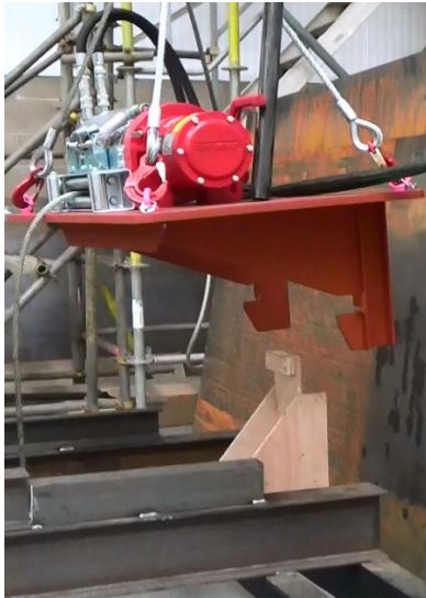
Fig. 17. Hydraulic Winch Deployment
