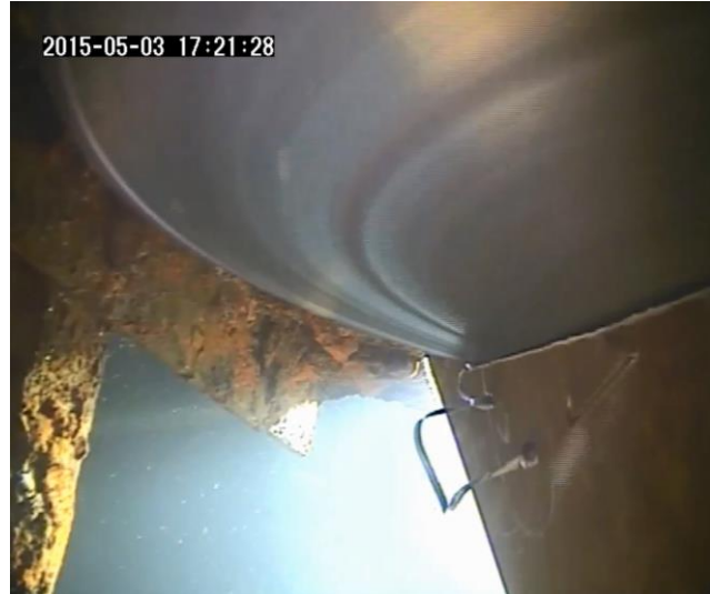
Fig. 13. Chute Cutting in PFSP
