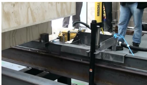
Fig. 4. Wheel Block Removal Tool Trial
