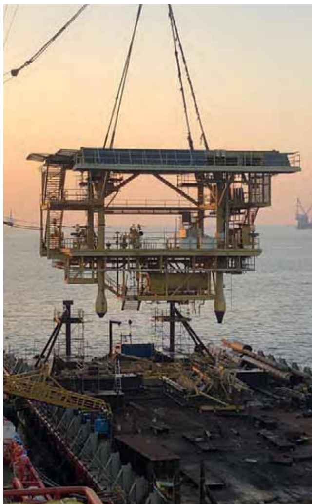
James Fisher Offshore decommissioning project in the Middle East
