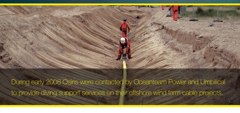
The first of these was the export cable replacement project undertaken at Scroby Sands OWF. The project called for the highest specification in diving equipment and experienced personnel. Throughout the operation the divers worked around the clock to achieve the recovery, replacement and reburial of one of the three export cables.
