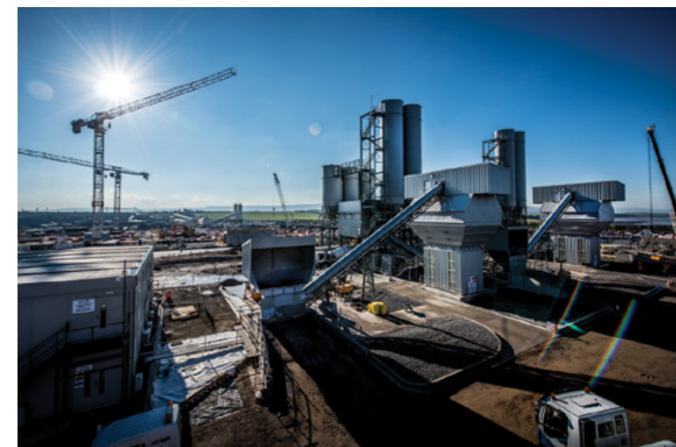
Hinkley Point C nuclear power station under construction
