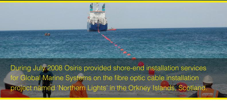
Osiris provided several dive teams and dive support vessels to conduct cable route video inspections, sink and position the cable on the seabed, conducted 1,400 metres of in-water burial, used divers to install articulated piping, drilled and affixed subsea anchor brackets and produced the "as laid position reports".
